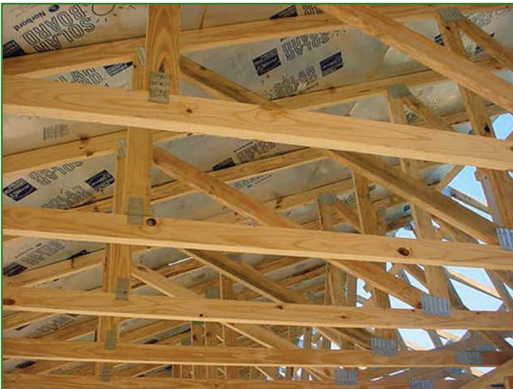
UHDC used radiant barrier sheathing to help insulate this home in Arkansas.
