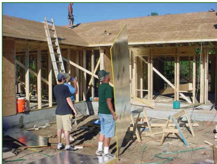
Aluminum sheathing reflects radiant heat away from the home and prevents solar heat gain, especially through the roof.
