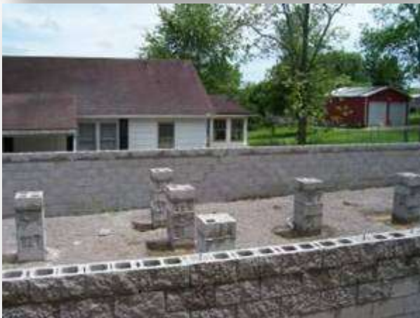
Solid Footers and Foundations
